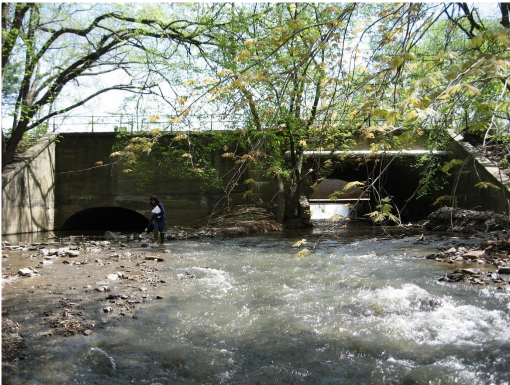
Downstream Headwall of Culvert (L) and Aqueduct (R) (Looking Upstream) – 2005
