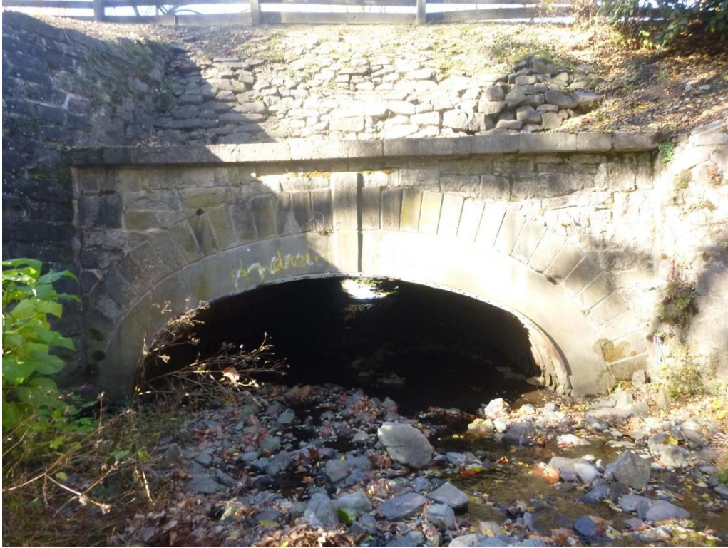
Upstream Headwall of Culvert (Looking Downstream) – November 5, 2025
