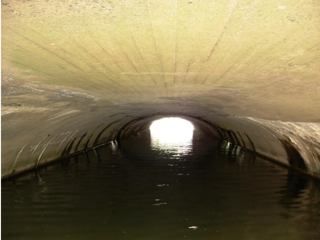
Inside Culvert (Looking Upstream) – 2007
