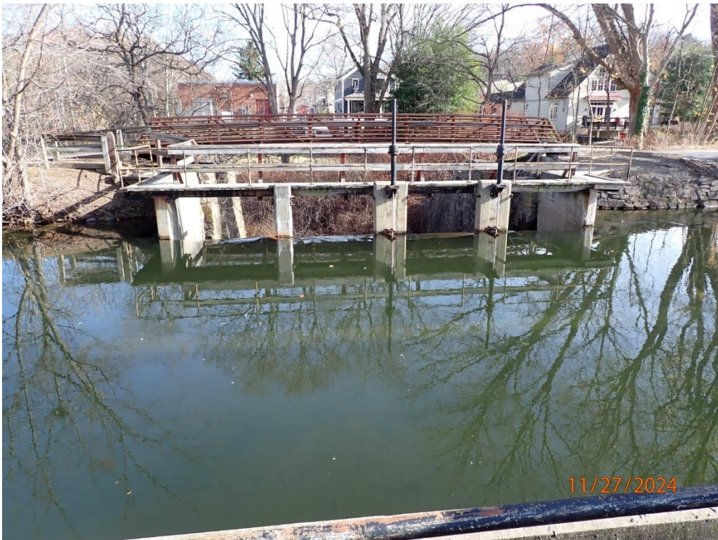
Aqueduct Canal Spillway – 2024
