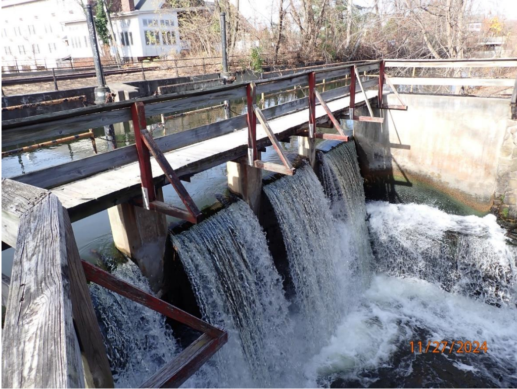
Aqueduct Canal Spillway – 2024
