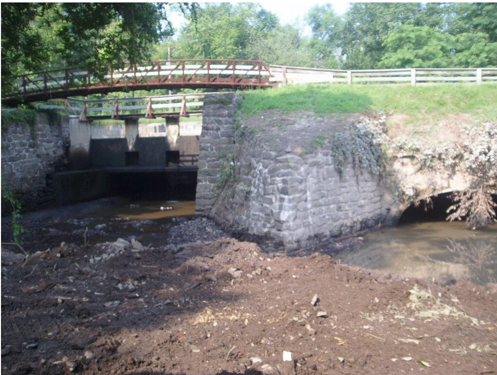
Upstream View of Aqueduct (L) and Culvert Headwall (R) (Looking Downstream) – 2005
