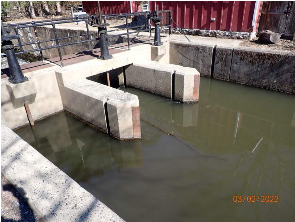
Photo 1: Griggstown Lock upstream side.
