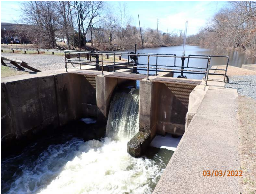
Photo 7: South Bound Brook downstream side.
