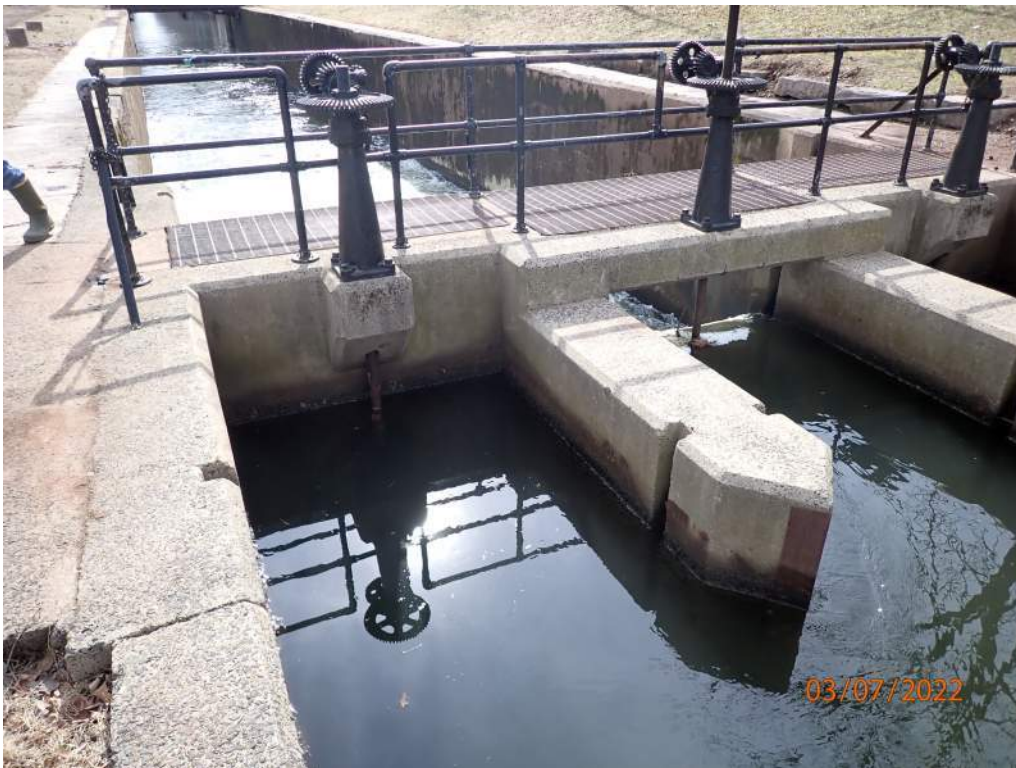
Photo 8: 5 Mile Lock upstream side.
