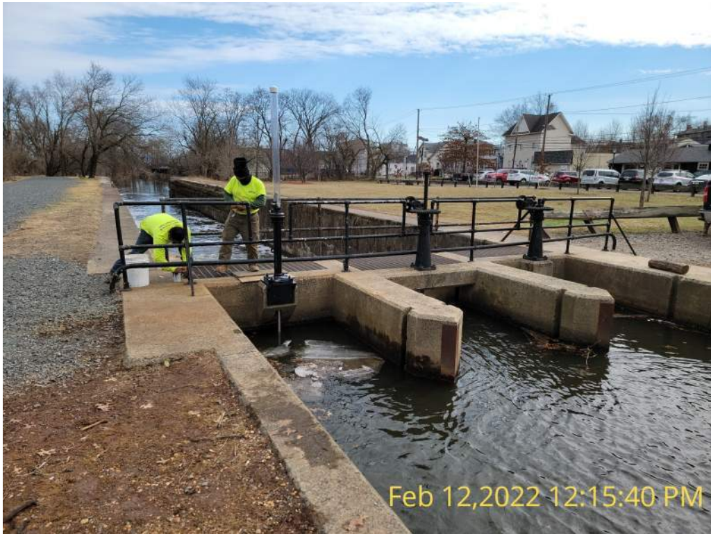
Photo 5: South Bound Brook upstream side.
