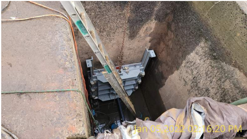
Photo 6: South Bound Brook lock left sluice gate work area dewatered.
