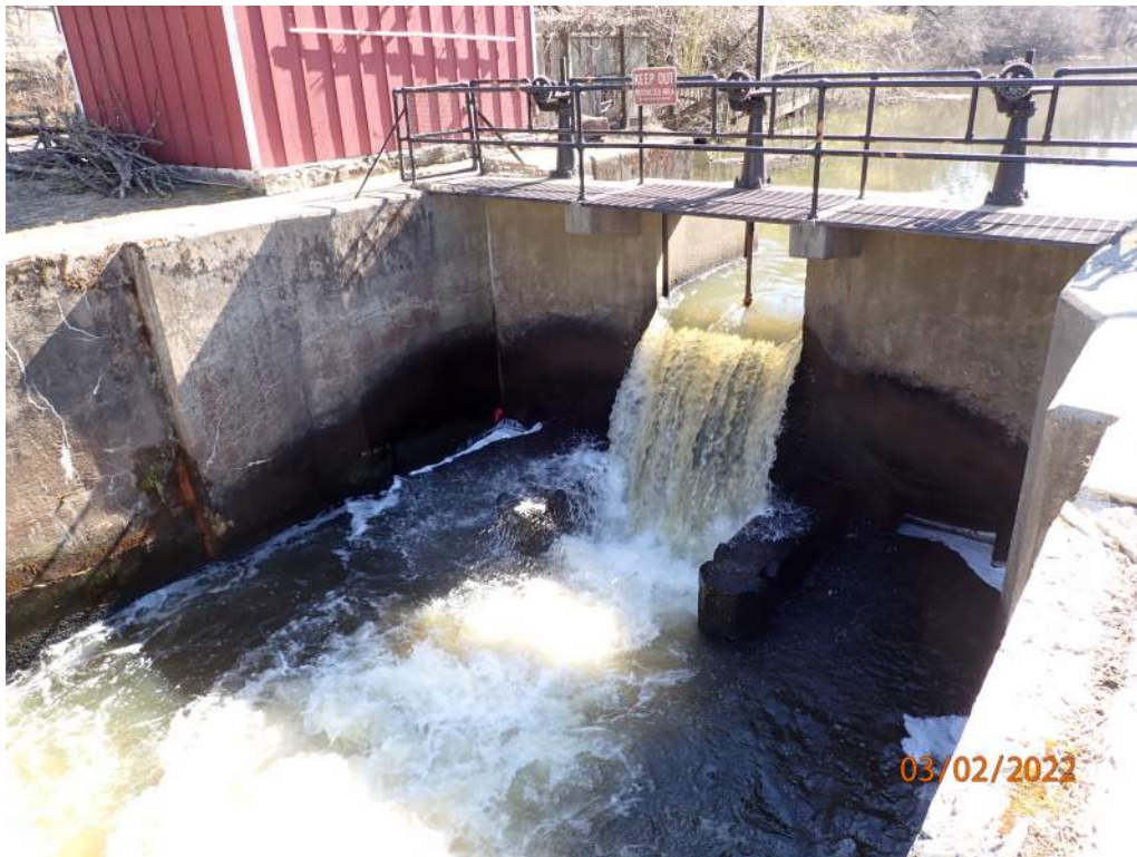
Photo 2: Griggstown Lock downstream side.
