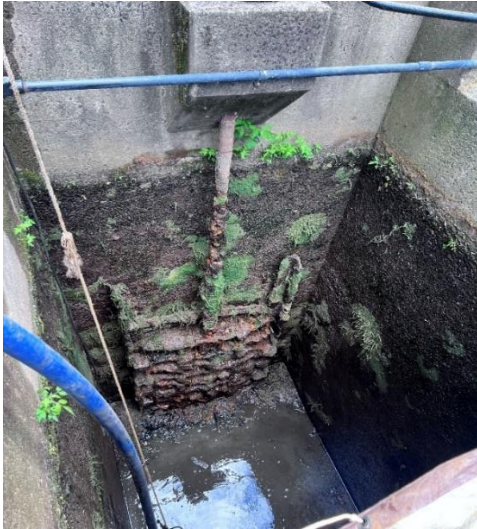
Original sluice gate in dewatered lock
