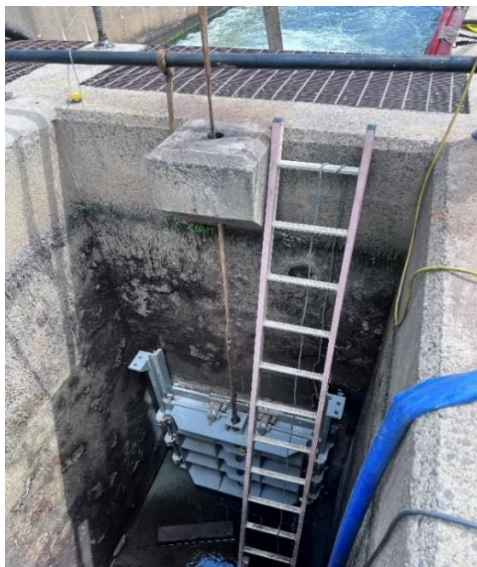
Replacement sluice gate
