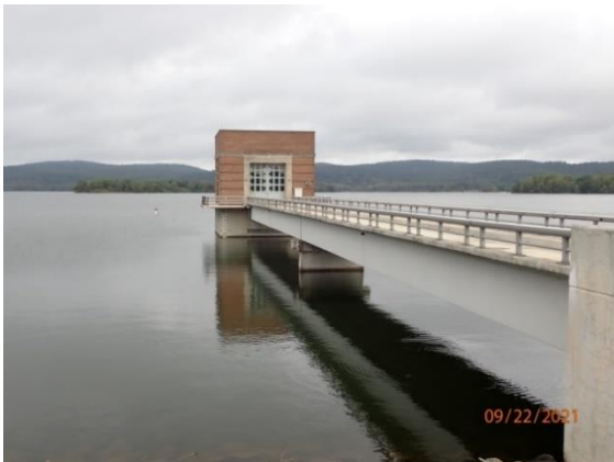
Spruce Run Reservoir's Tower and Access Bridge
