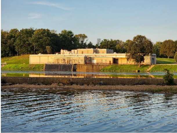
South Branch Pump Station
