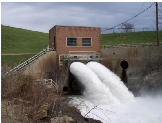
Spruce Run Reservoir's Outlet Vault
