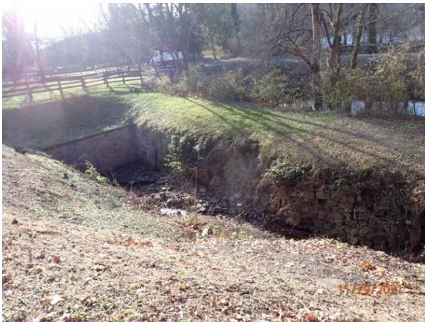
Existing condition of the Prallsville Culvert Pit.
