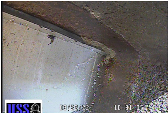
Epoxy holding rubber seal in place
