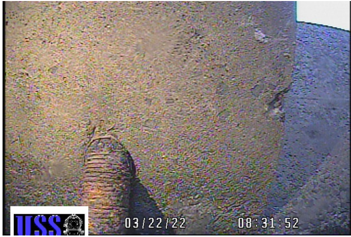
Operating stem passing through concrete
