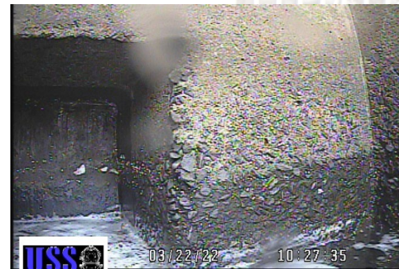
Condition of bulkhead downstream of gate
