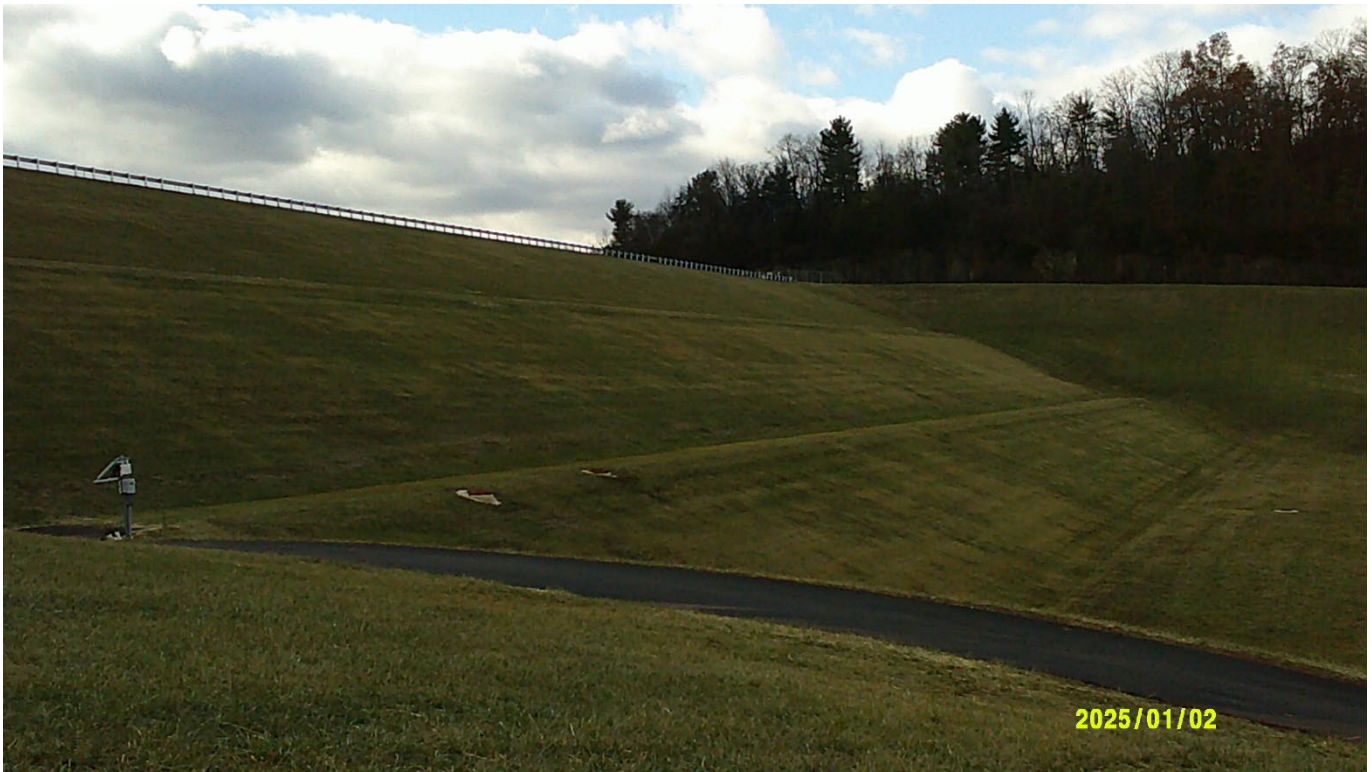
Completed North Dam Embankment Work.
