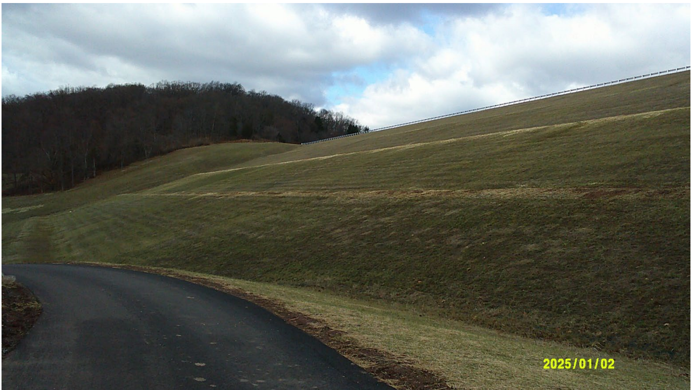
Completed South Dam Embankment Work.
