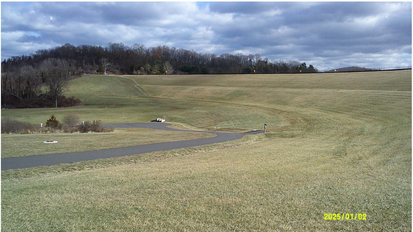
Completed Dike Embankment Work.
