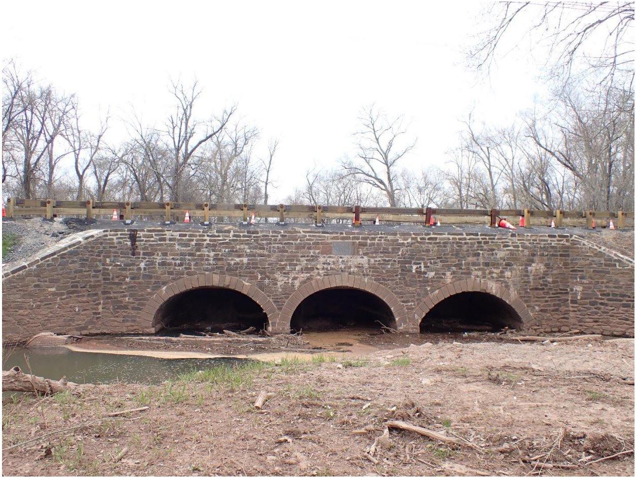
View of Culvert Inlet. Repointed stonework on headwall and within culvert. Repaved, restriped, and new guiderail installed on Canal Road (above)
