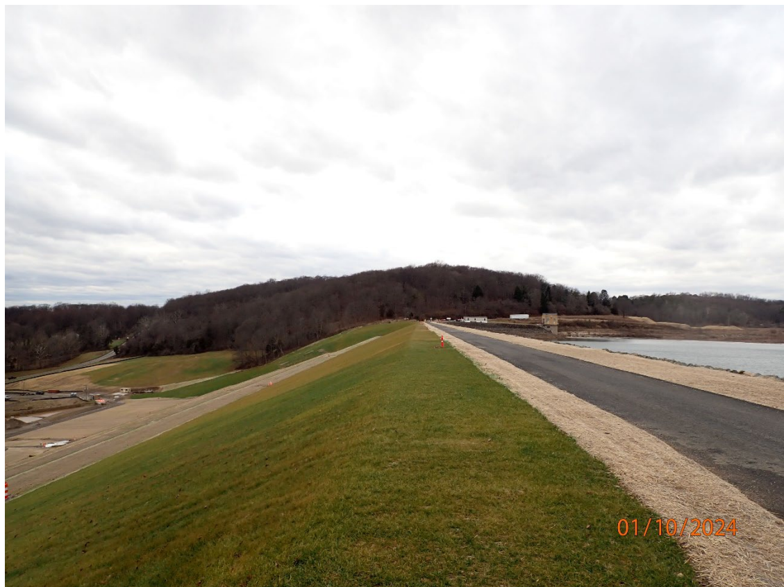
Crest of the South Dam – General View
