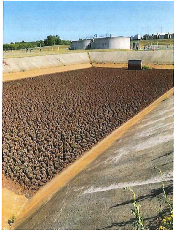
Improved residuals drying from lagoon drainage and piping repairs
