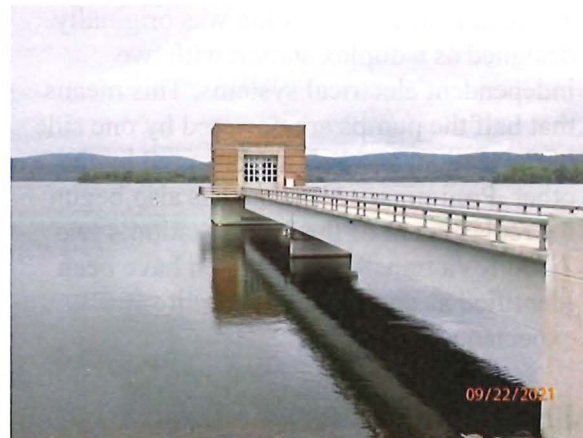
Spruce Run Reservoir's Tower and Access Bridge
