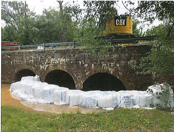
Cofferdam installed at Six Mile Run Culvert.
