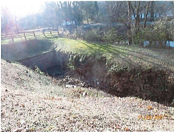
Existing condition of the Prallsville Culvert Pit.
