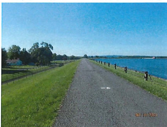
Spruce Run Reservoir Dam SE View from Sta. 5+50
