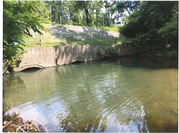
Six Mile Run Culvert (West Headwall)
