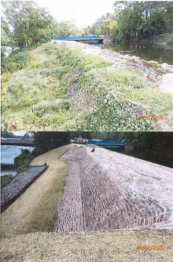
Landing Lane Spillway before (top) and after (bottom) the 2022-2023 rehabilitation project.
