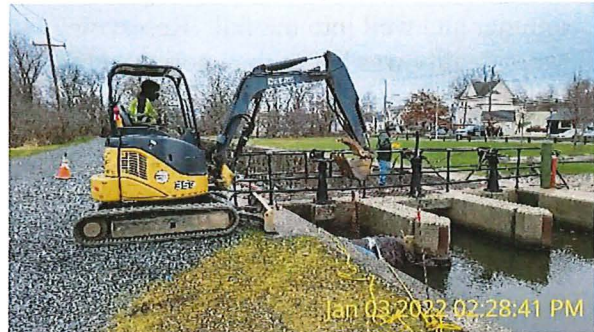
Emergency sluice gate replacement at South Bound Brook Lock
