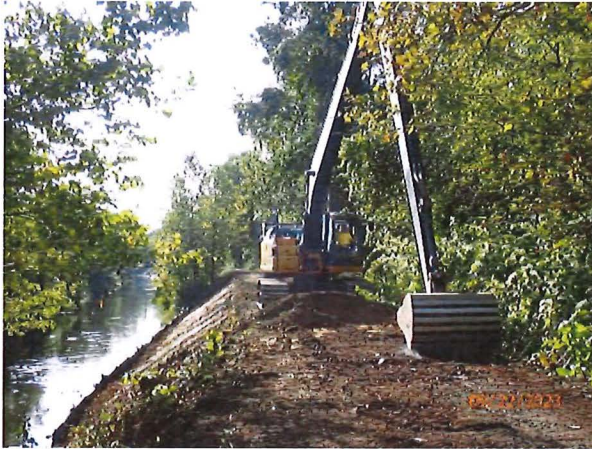
Restoration of the Canal embankment in Stockton
