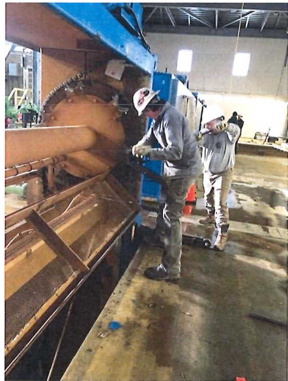
Traveling water screen repair work
