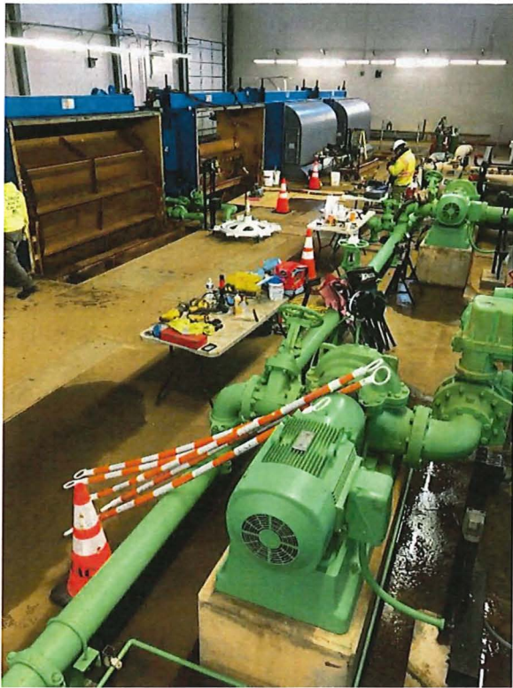
Traveling water screen repair work
