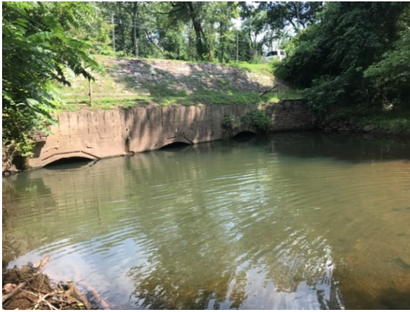
Six Mile Run Culvert (West Headwall )
