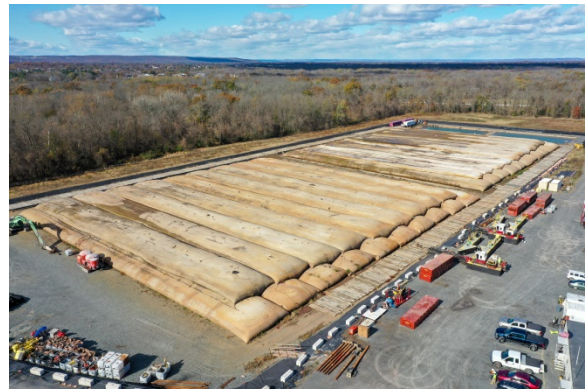
The sediment dewatering site during operations
