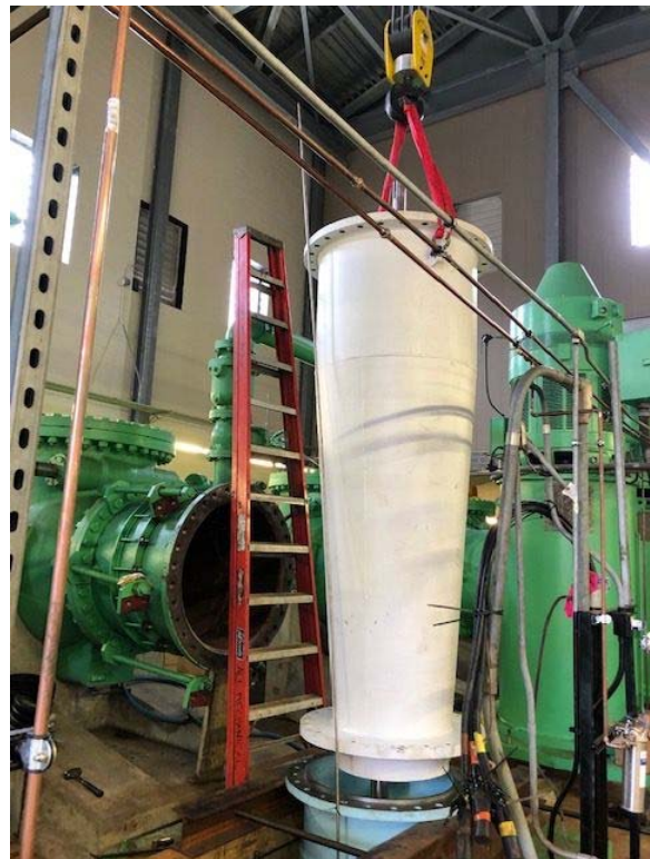
Reassembly of the intake pump
