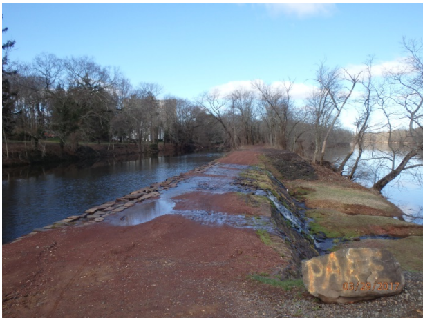
Crest of the Landing Lane Spillway
