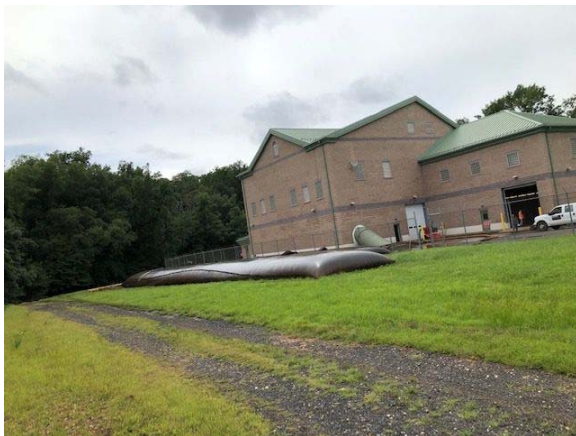
Geobag used to dewater sediment at intake pump station
