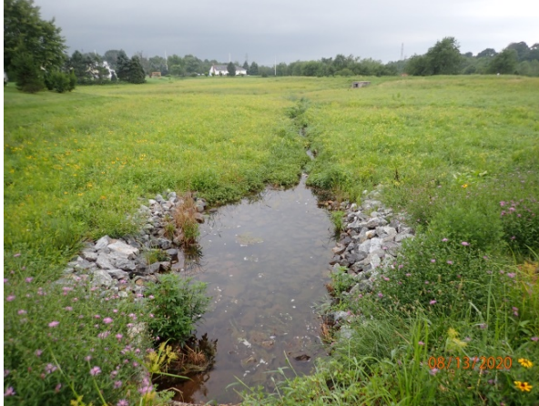
Laird Terrace Stormwater Detention Basin after modifications to improve water quality
