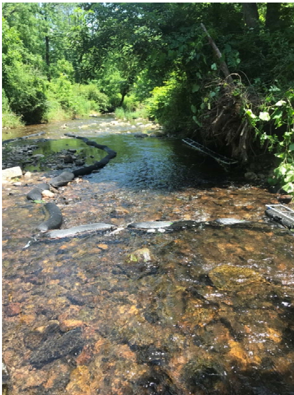
Mulhockaway Creek Biochar Installation, June 2021
