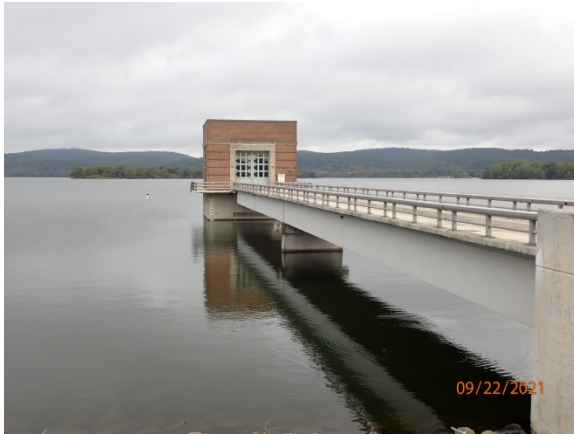
Spruce Run Reservoir's Tower and Access Bridge
