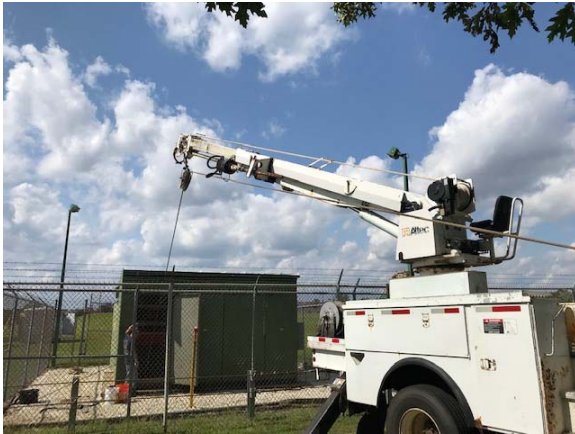
High voltage cable replacement
