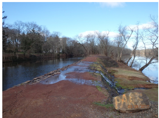
Crest of the Landing Lane Spillway.
