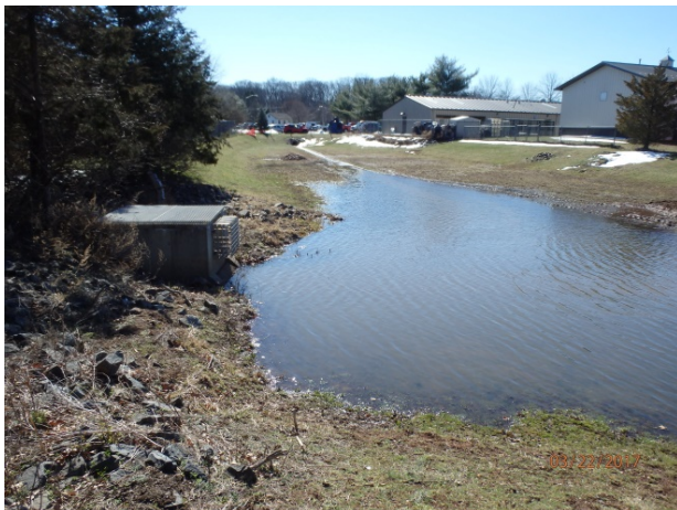
Municipal Complex Stormwater Detention Basin.
