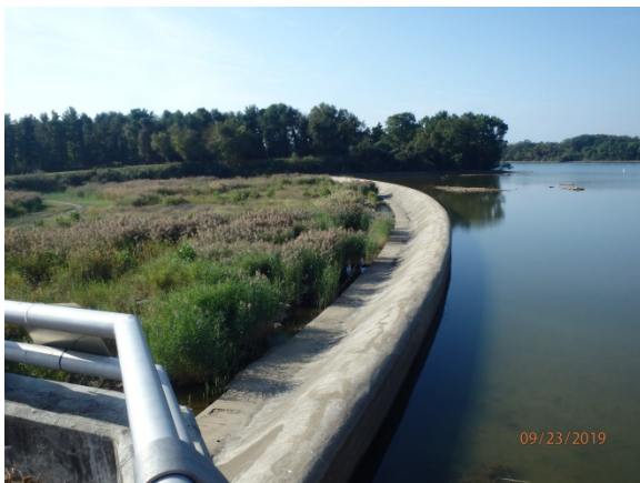
Spruce Run Reservoir Primary Spillway.
