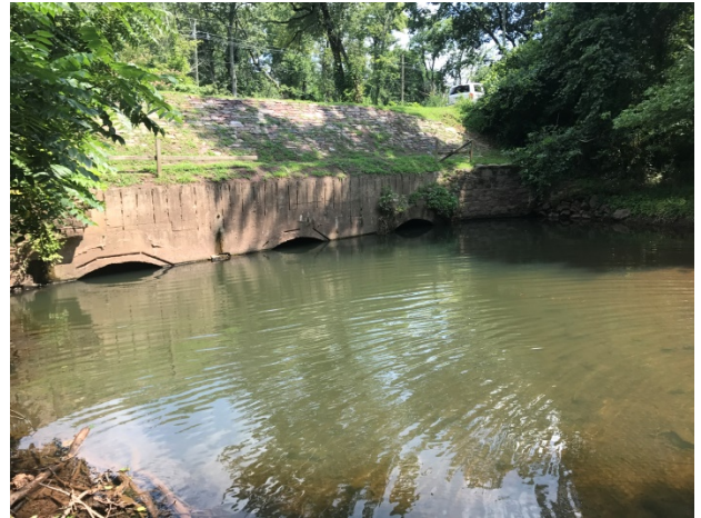
Downstream side of Six Mile Run Culvert.
