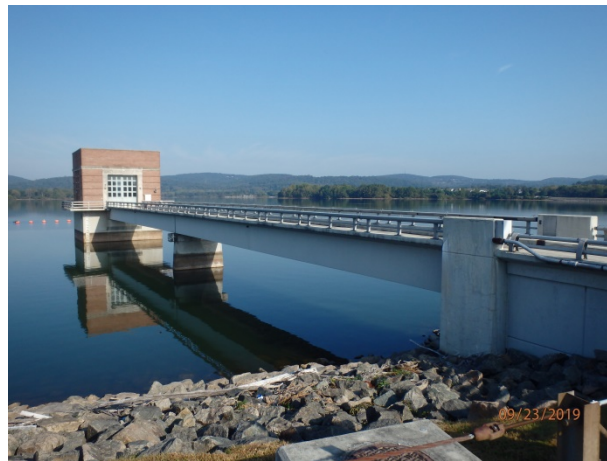
Spruce Run Reservoir Inlet/Outlet Tower
