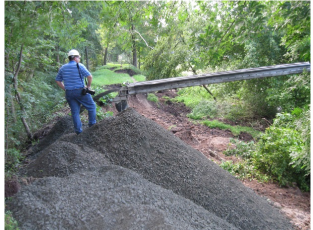
Placement of DGA by conveyor across the Canal.
