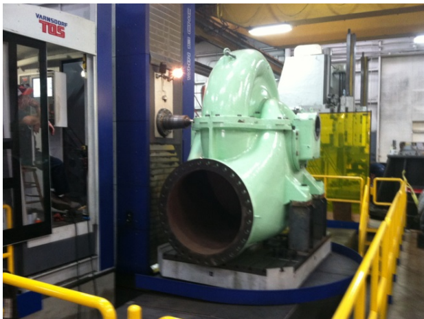
South Branch Pump Station 2000-HP pump under rehabilitation.
