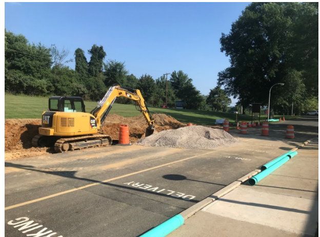
Spruce Run Administration Building emergency sewer pipe replacement.
