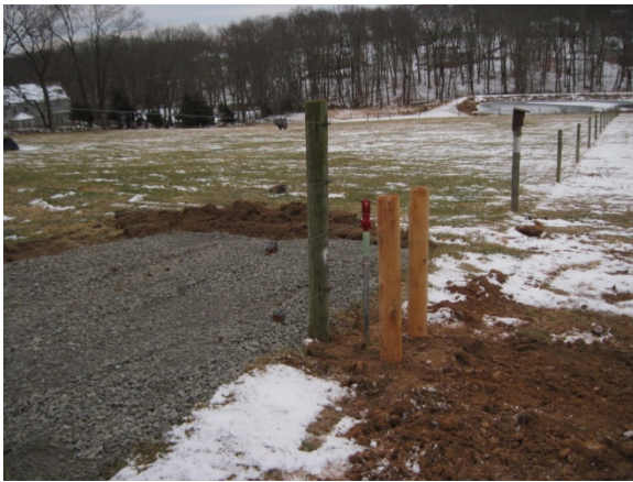
Heavy use area protection at a farm participating in the RCPP program. This project will help reduce soil erosion and sediment transport into nearby waterways.
