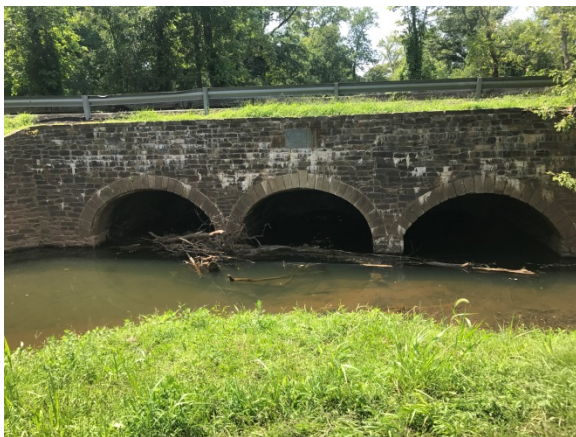
Upstream side of Six Mile Run Culvert.
