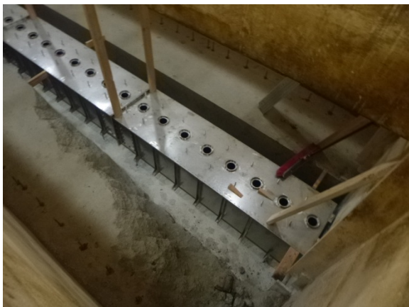
Underdrain reconstruction at the MWTP
