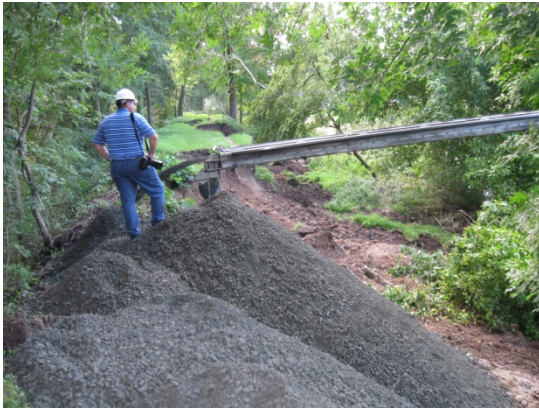
Placement of DGA by conveyor across the Canal.
