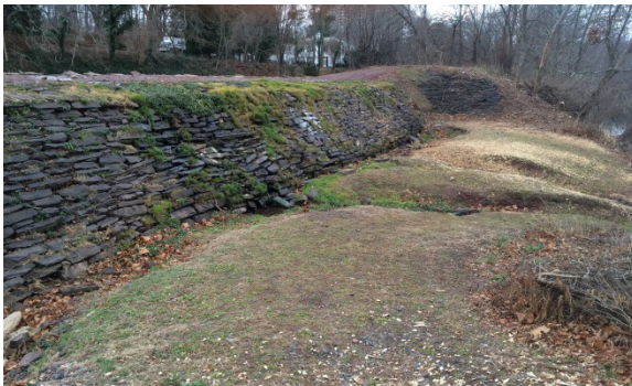
River side slope of Landing Lane Spillway.
