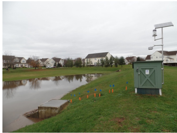
Pre-retrofit monitoring of the Renoir Detention Basin in Franklin Township, Somerset County
