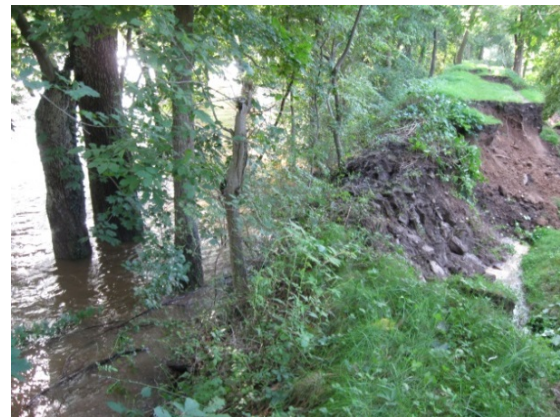
D&R Canal embankment in Stockton Borough in 2011.
