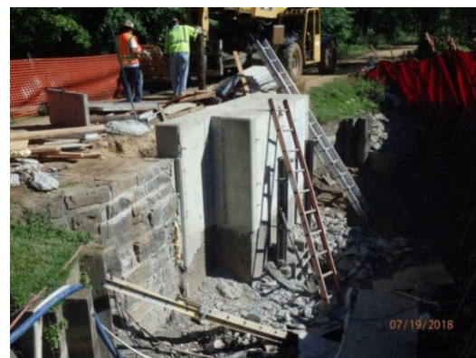
Griggstown Waste Gate. New concrete placed in upper part of structure.
