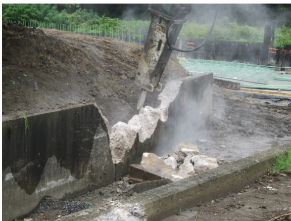
Demolition work at Cherry Tree Lane Spillway.
