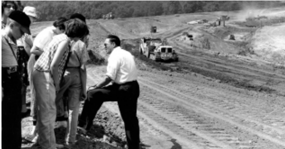
Construction of Round Valley Reservoir in the 1960s.
