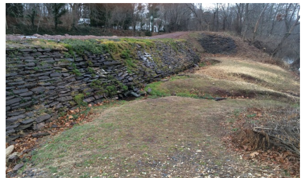
River side slope of Landing Lane Spillway.
