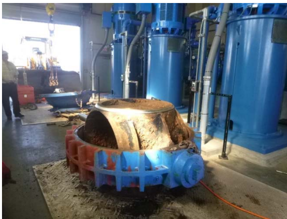
Large Valve Repair work.
