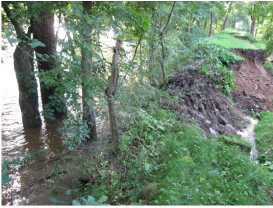
D&R Canal embankment in Stockton Borough in 2011.
