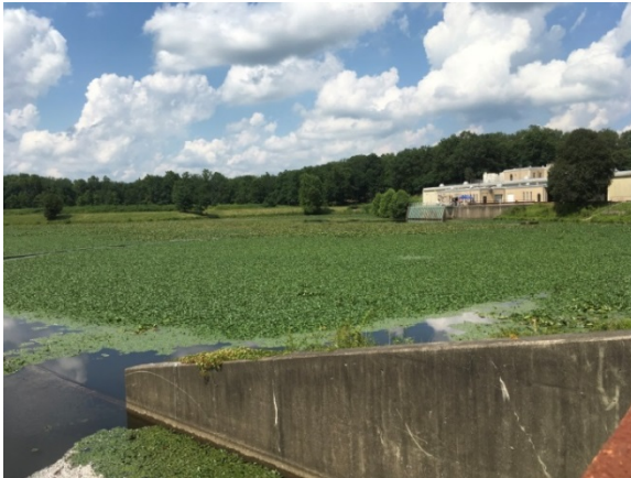
South Branch Pumping Station, August 2017
