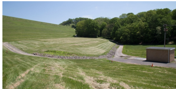
Round Valley South Dam and vault
