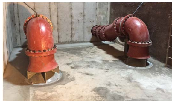
Wall and new internal piping.
