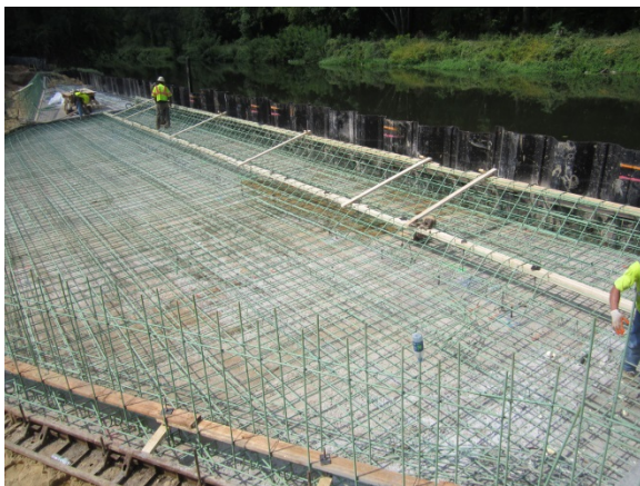
Reinforcing steel before concrete pour at Cherry Tree Lane Spillway
