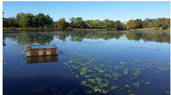
South Branch Pumping Station Intake Pond
