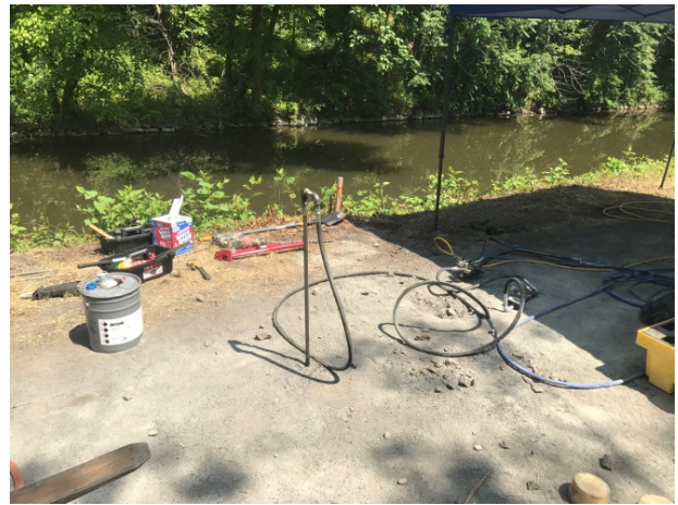
West Amwell seepage repairs. Chemical grout injection points. Canal in background.
