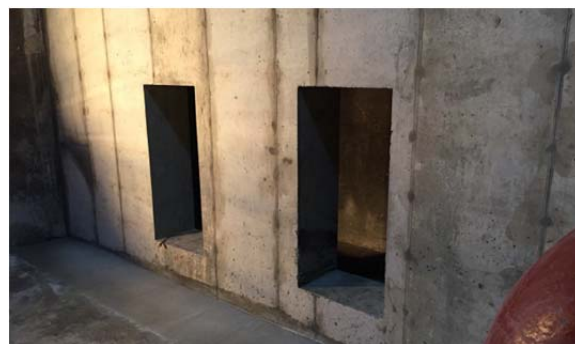
Wall and new internal piping.
