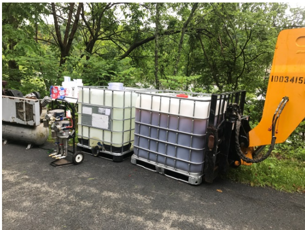
West Amwell seepage repairs. Chemical grout “totes.”
