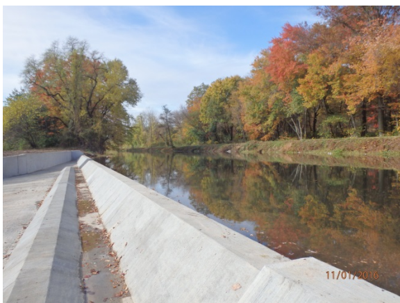
Completed Cherry Tree Lane Spillway.
