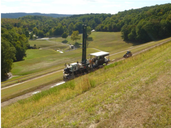
Drill rig installing new instrumentation on embankments
