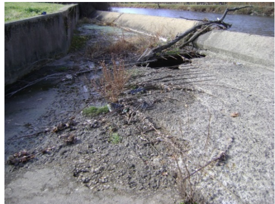
Cherry Tree Lane Spillway
