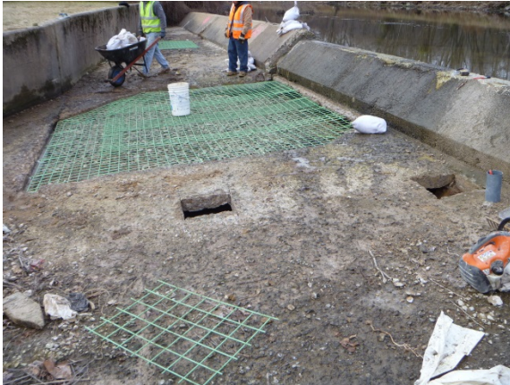
Emergency repair work at Cherry Tree Lane Spillway
