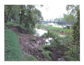
Partial failure of the western embankment in Stockton Borough, Hunterdon County following Tropical Storms Irene and Lee in 2011. Note level of the Delaware River relative the crest of the embankment and the seepage through the embankment. At the peak elevation, the river was only about six inches from overtopping certain sections of the embankment.
