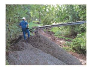
Pictured above is the placement of the DGA by conveyor across the Canal. The DGA was used to restore the embankment to prevent a breach. The DGA was compacted as conditions permitted and the crest of the embankment was covered with a liner to reduce erosion caused by precipitation.
